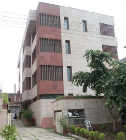
Spectra Services Consultants Office Building, Noida, Platinum rated
